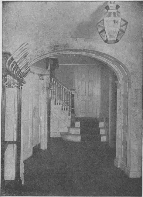
THE HALL AND STAIRCASE.
